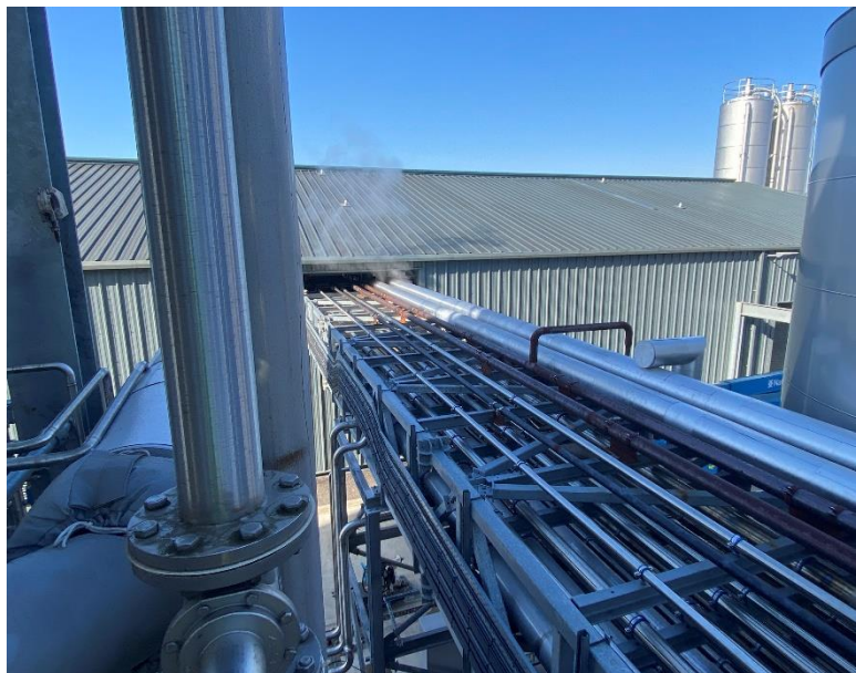
The pipe bridge which supports the pipework to convey the cooked media and inoculum to the large-scale fermenter vessels.
