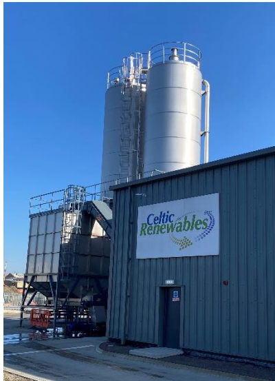
Draff and Potato storage hoppers operational at the front-end of the plant.
