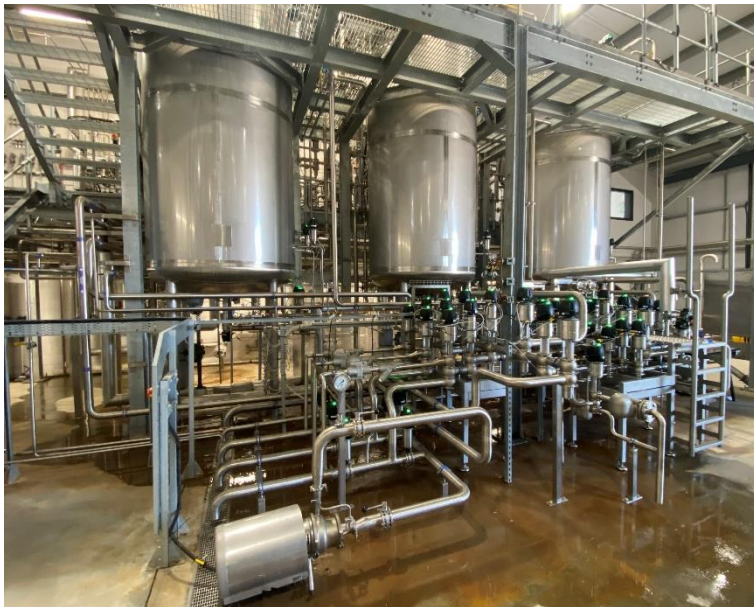
The 3 final stage 5,000l inoculum vessels have been operating reliably since Nov 2022, which feed the large-scale production fermenters, pictured above.
